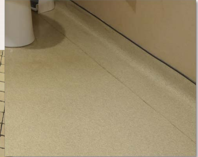
WORN SHEET VINYL WITH CURLING SEAMS
