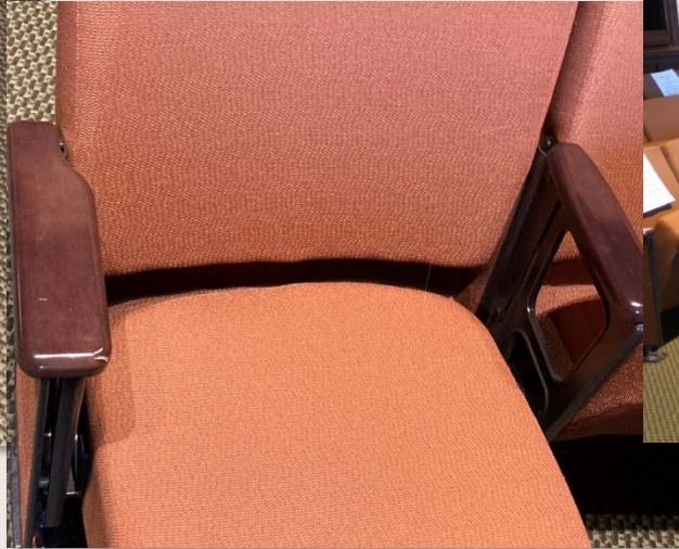
WORN CUSHIONS AND RETRACTION SPRINGS
