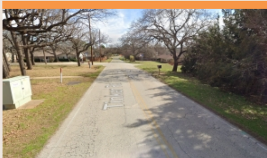
Looking East at Ponderosa Ln 21-foot wide existing section
