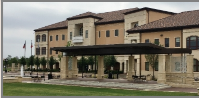
Plaza at City Hall Contract Award $2,774,547 Final Contract Cost $2,772,837
