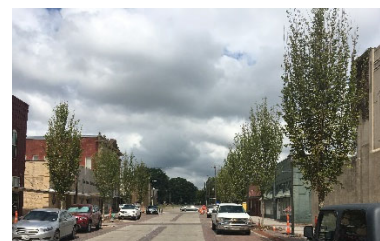
Recently installed streetscape
