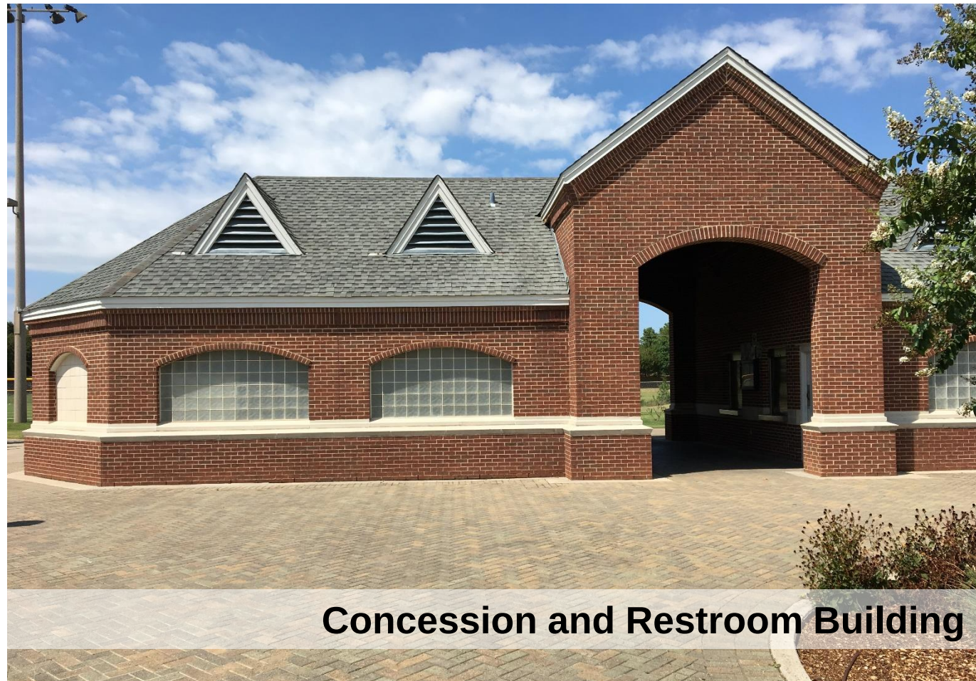
Existing Concession and Restroom building renovated
