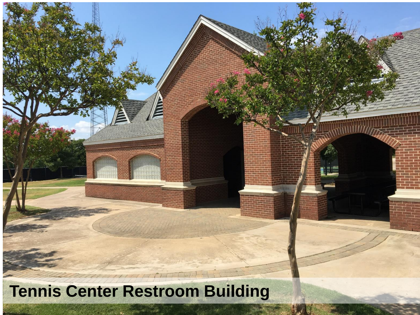
Existing Tennis Center restroom building renovated
