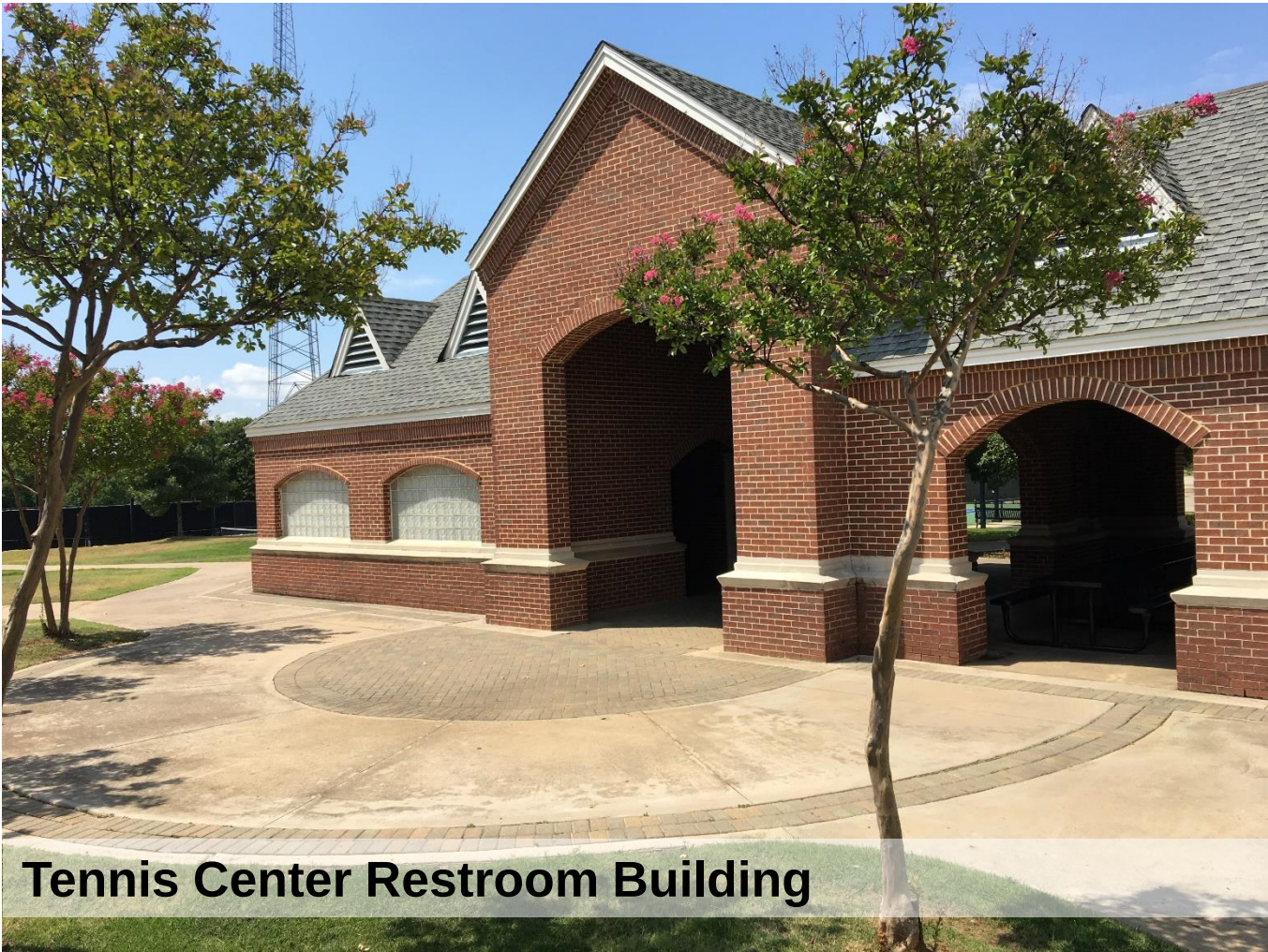
Existing Tennis Center restroom building renovated
