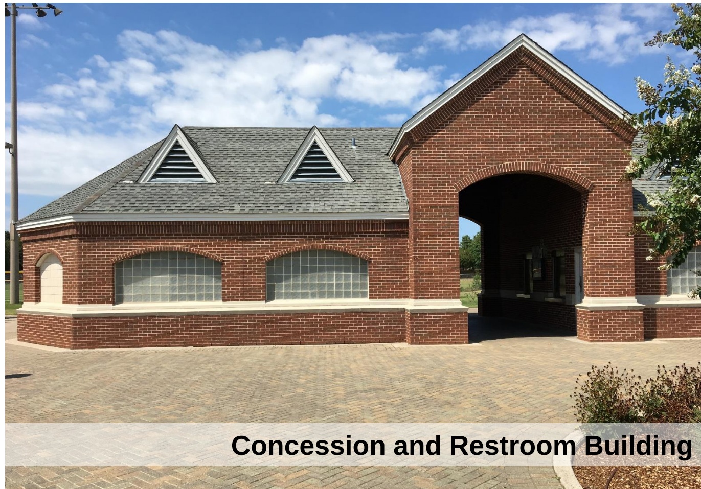
Existing Concession and Restroom building renovated
