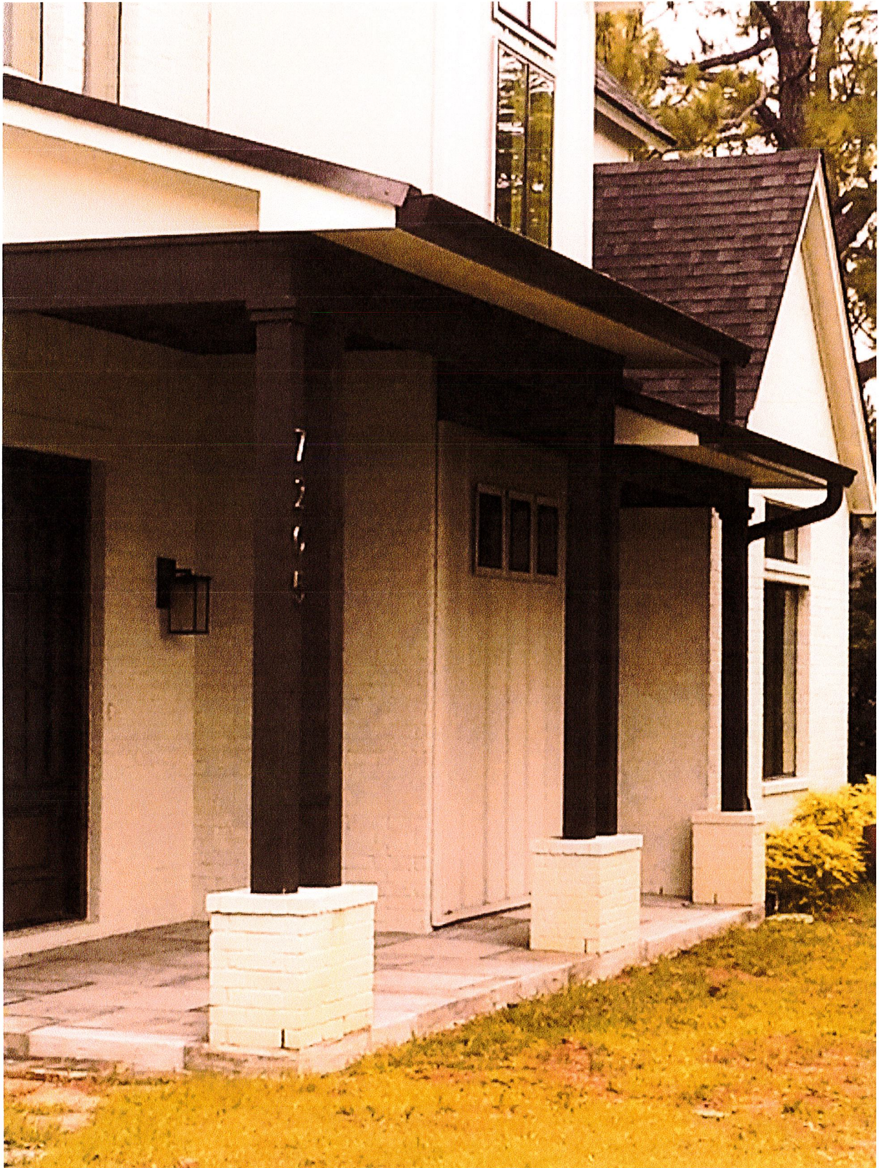
EXISTING MAIN DWELLING – FRONT PORCH COLUMN DETAIL
