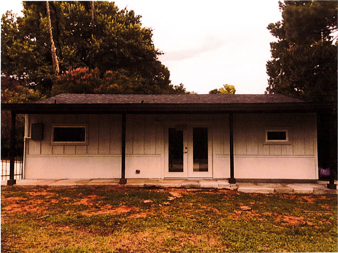
EXISTING ACCESSORY DWELLING – COVERED FRONT PORCH ELEVATION
