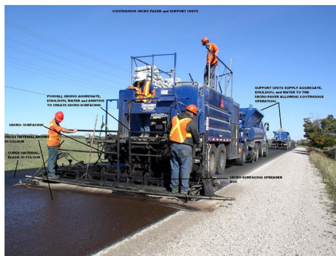
Figure 4: Application of Micro-Resurface
