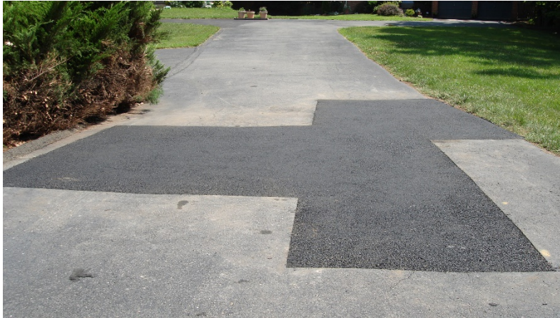
Figure 5: Asphalt Base Repairs
