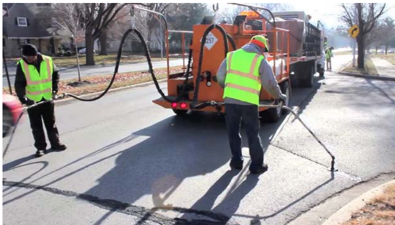
Figure 6: Application of Crack Sealing
