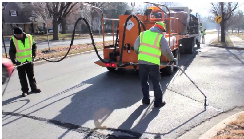
Figure 6: Application of Crack Sealing
