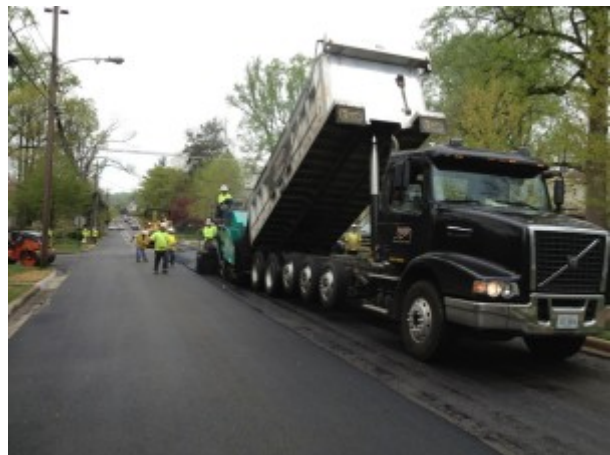
Figure 2: Asphalt Placement
