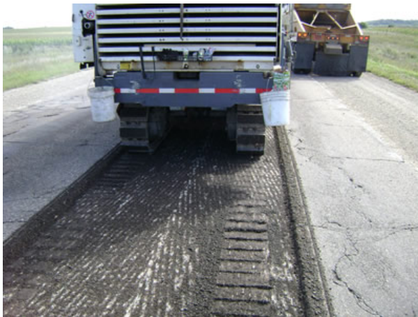
Figure 1: Milling
