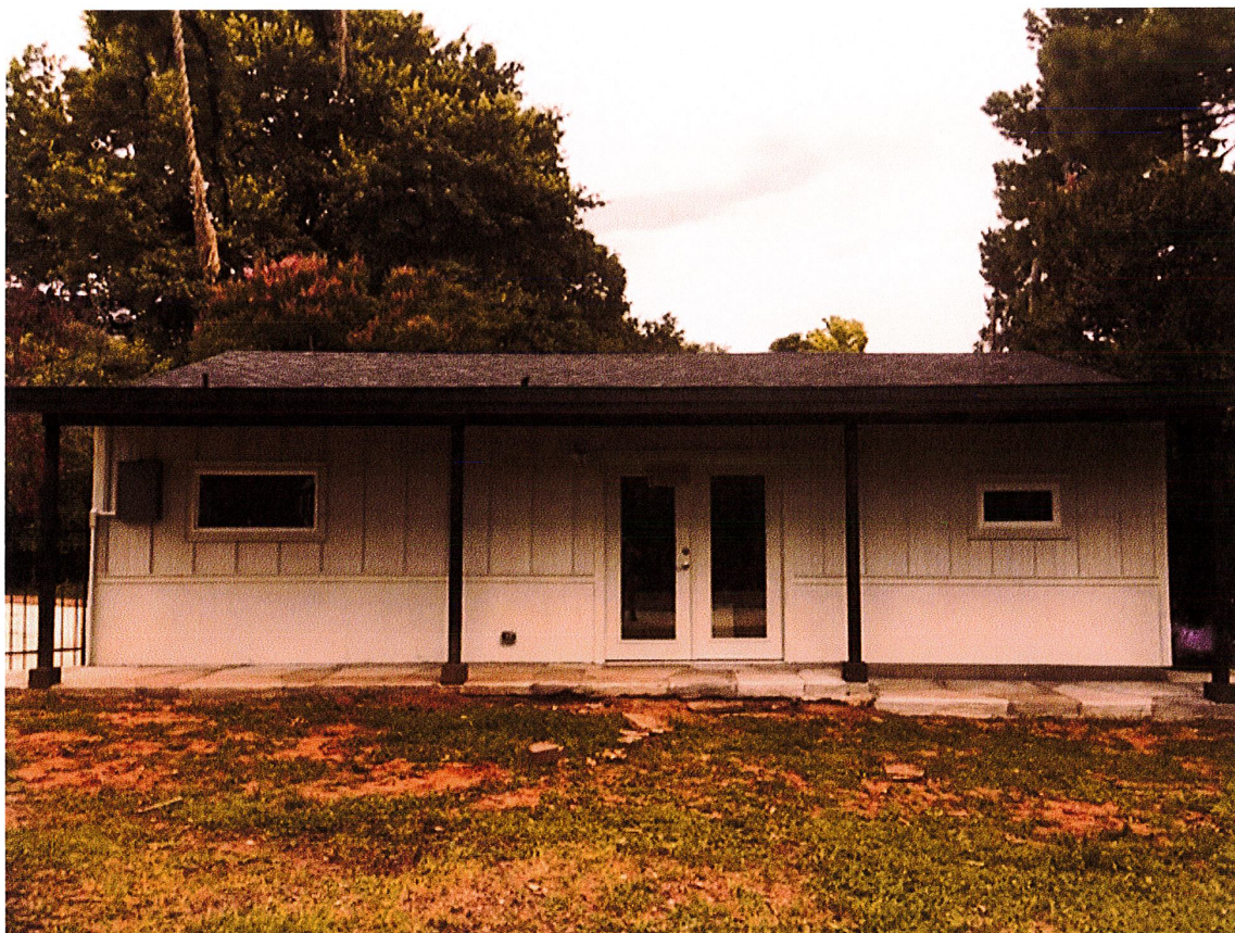
EXISTING ACCESSORY DWELLING – COVERED FRONT PORCH ELEVATION
