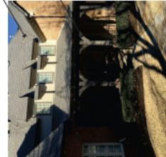
7 PHOTO OF EXISTING HOUSE
