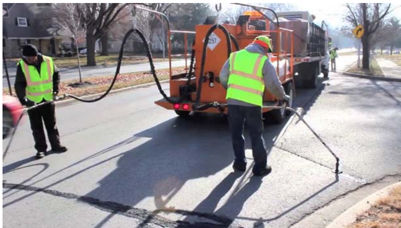
Figure 6: Application of Crack Sealing
