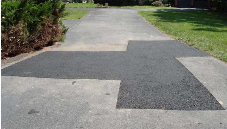
Figure 5: Asphalt Base Repairs
