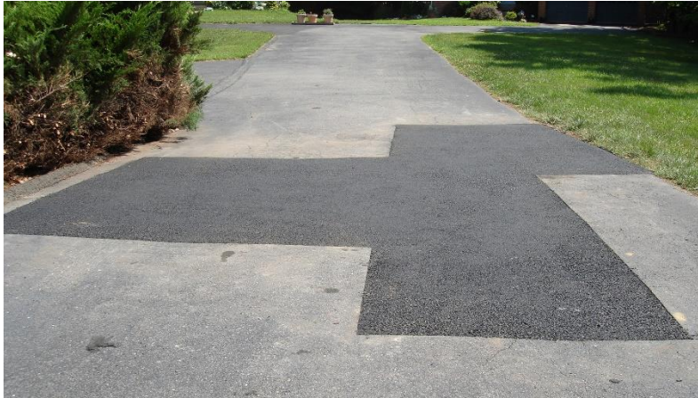
Figure 5: Asphalt Base Repairs
