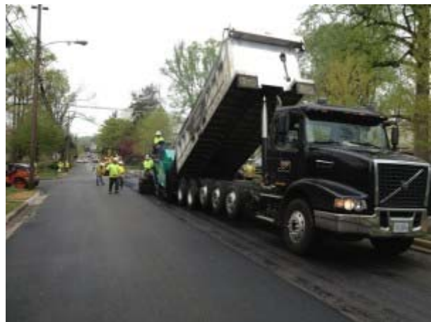
Figure 2: Asphalt Placement
