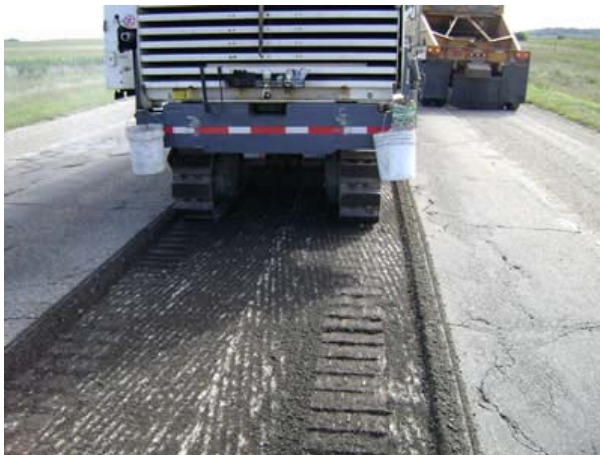
Figure 1: Milling
