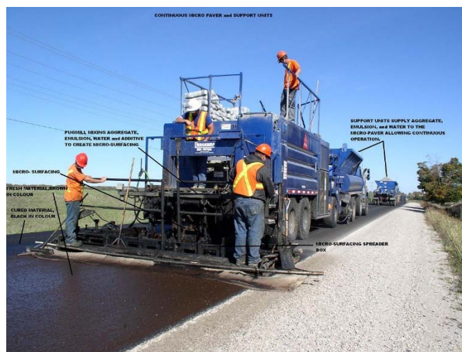
Figure 4: Application of Micro-Resurface
