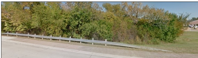
# 51 Vacant Land (Drainage Area) 4520 Colleyville Blvd.
