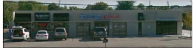
# 12 Multi-Tenant 3919 Colleyville Blvd.
