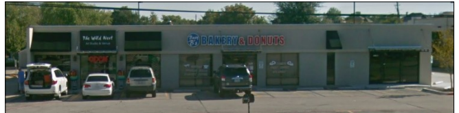
# 12 Multi-Tenant 3919 Colleyville Blvd.
