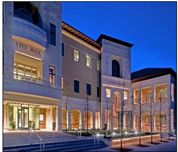
Colleyville City Hall
