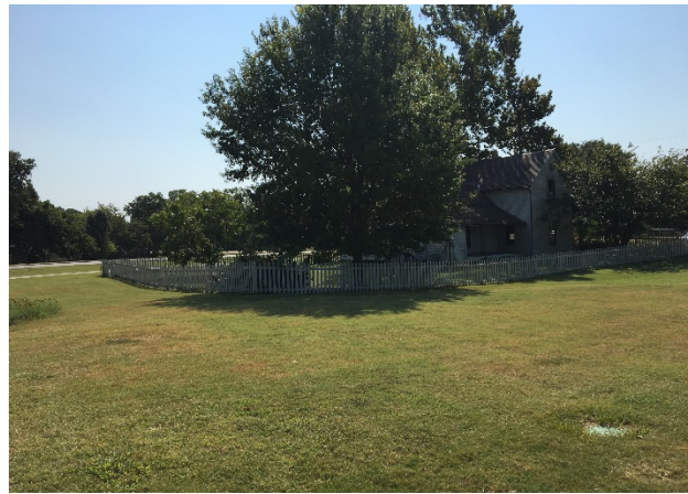
North and west facades
