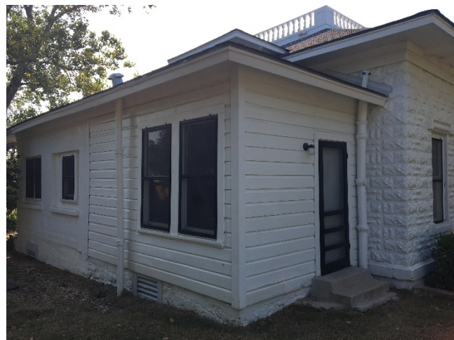
The existing structure includes a single-story addition on the north. The addition is not constructed of the cast concrete block.
