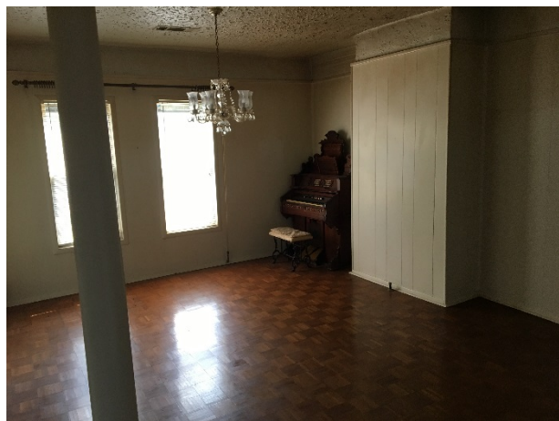
Existing dining room configuration
