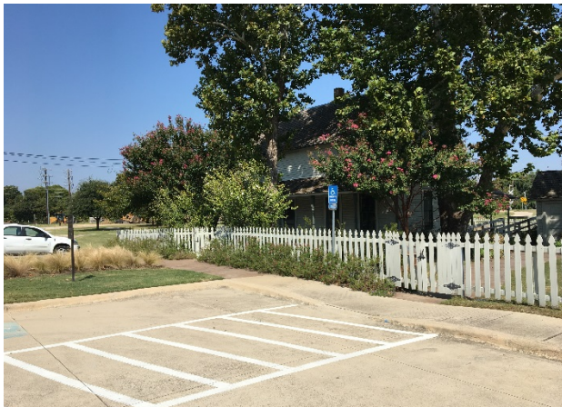
South façade and Handicap parking
