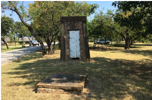
Existing well and pump house
