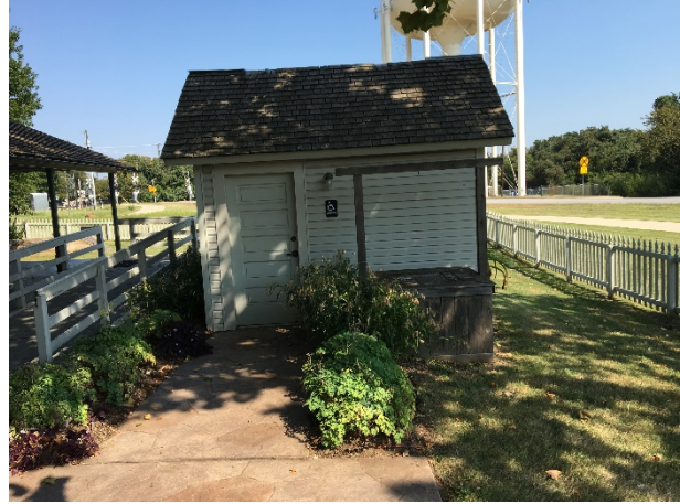
Existing ramp and restroom
