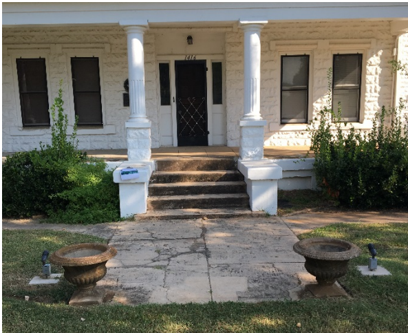
The existing first floor is raised above the existing grade
