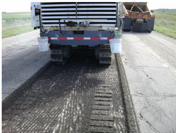
Figure 1: Milling
