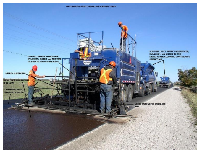
Figure 4: Application of Micro-Resurface
