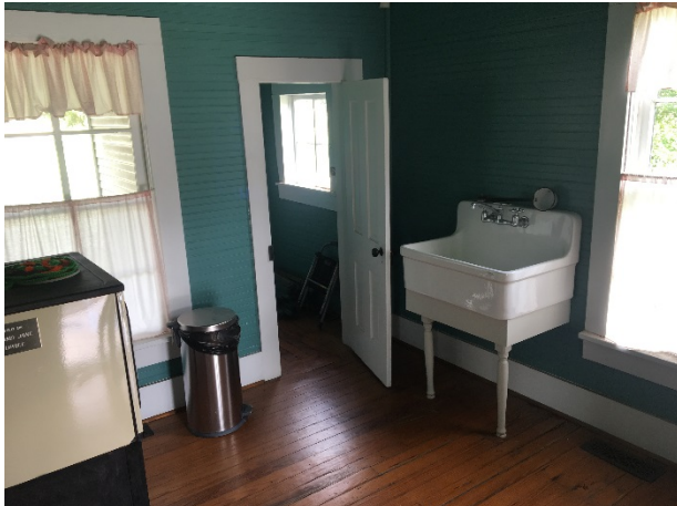
Existing kitchen configuration
