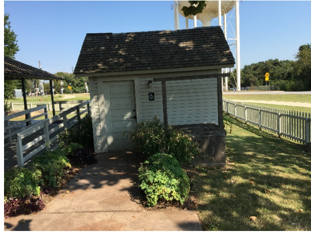
Existing ramp and restroom
