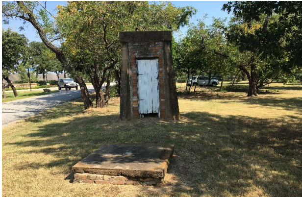
Existing well and pump house
