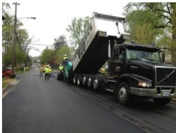
Figure 2: Asphalt Placement
