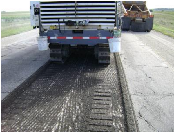
Figure 1: Milling
