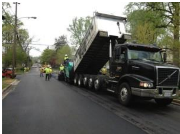
Figure 2: Asphalt Placement
