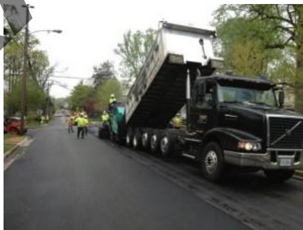
Figure 2: Asphalt Placement
