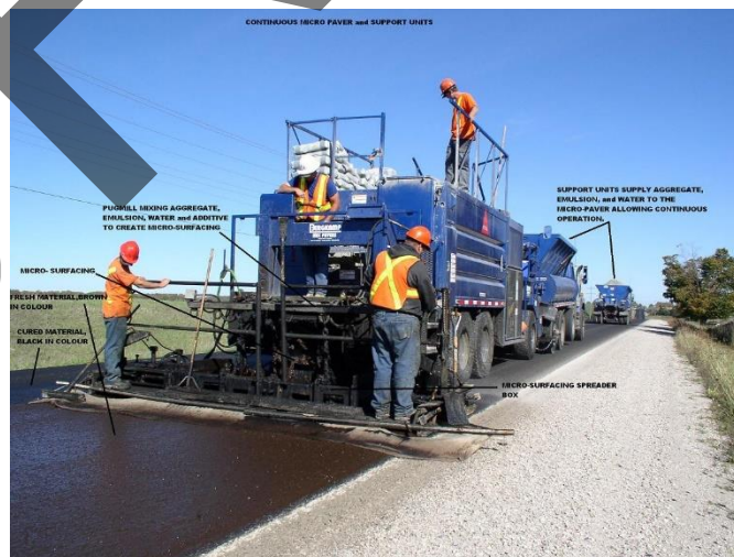
Figure 4: Application of Micro-Resurface
