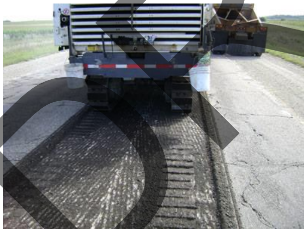
Figure 1: Milling
