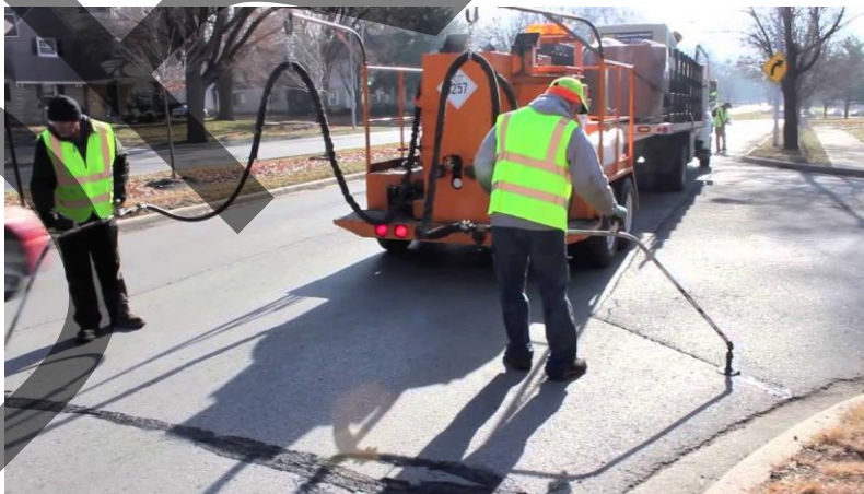
Figure 6: Application of Crack Sealing
