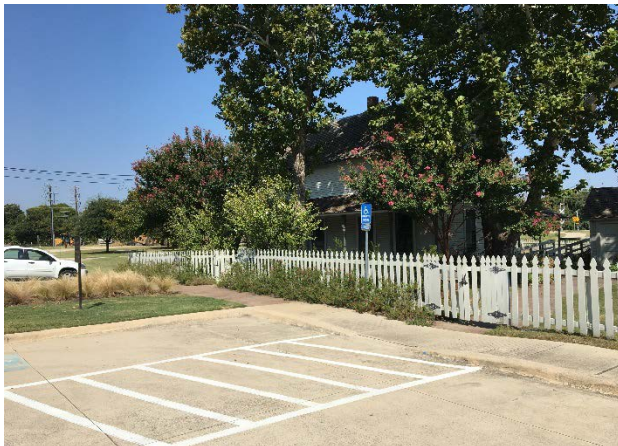
South façade and Handicap parking
