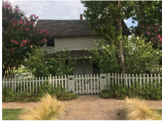
Webb House exterior entry
