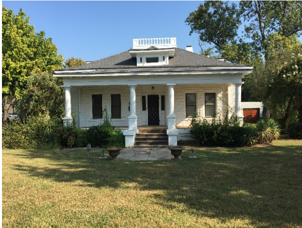
Front Façade of Bidault House
