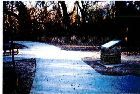
Path intersections should be clear and open like this to help ensure avoidance of traffic conflicts.
