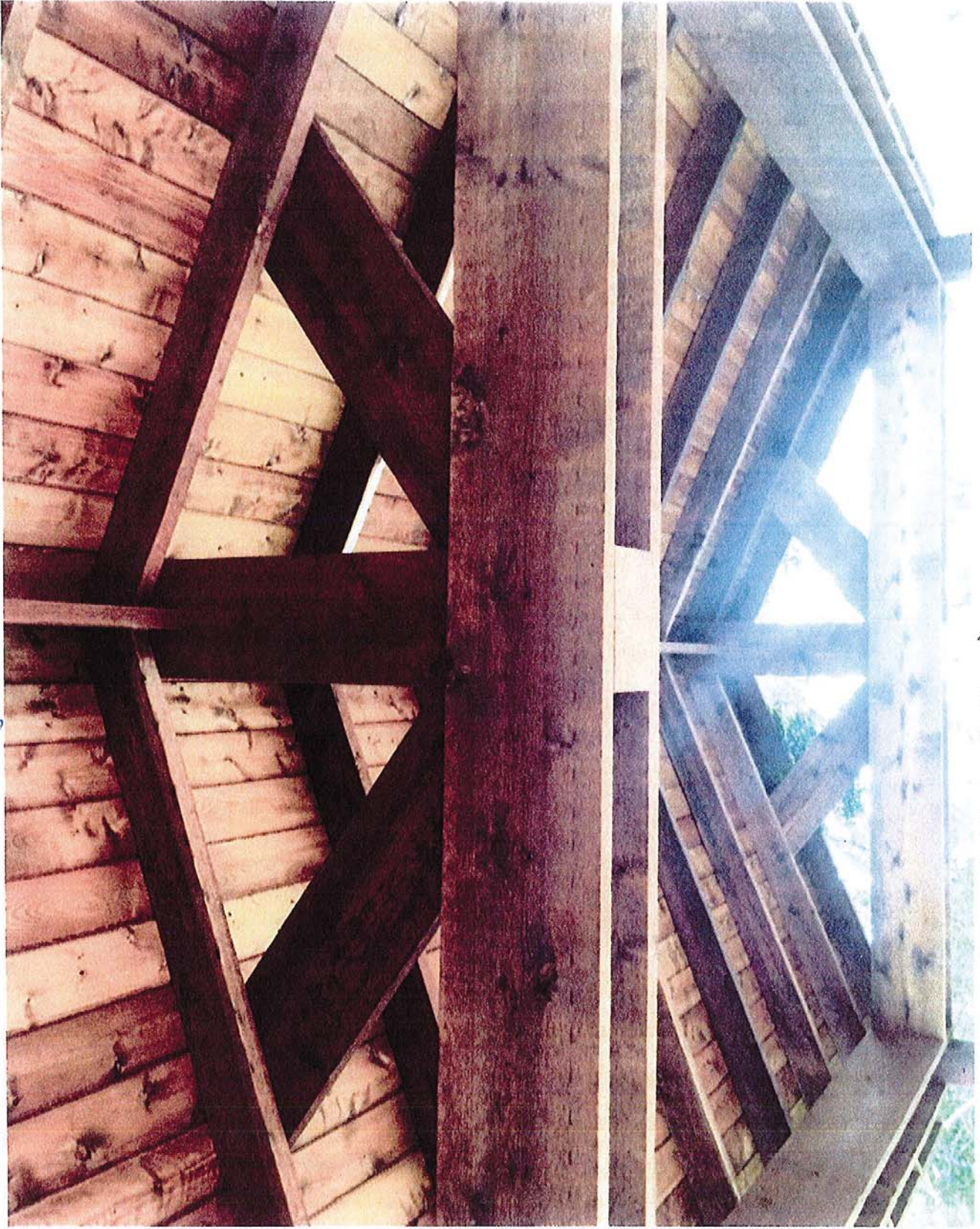
under gable roof structure
