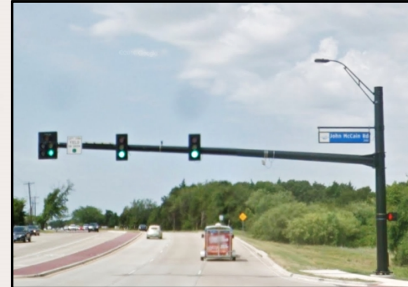
Powder Coated Signal Poles
