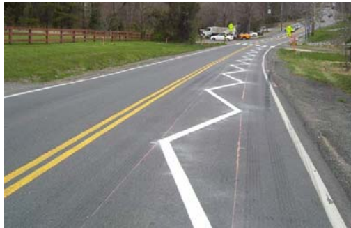
Figure 2: Zig-Zag Pavement Marking Example 2
