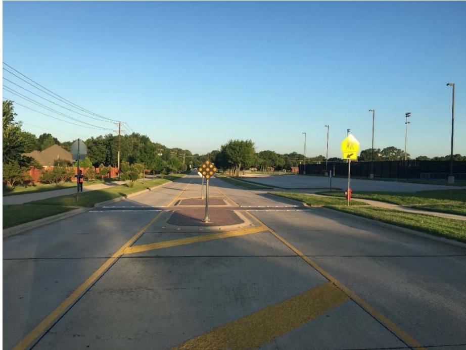
Location 8: Bogart Dr. at west of Hidden Oaks Dr., Westbound Approach
