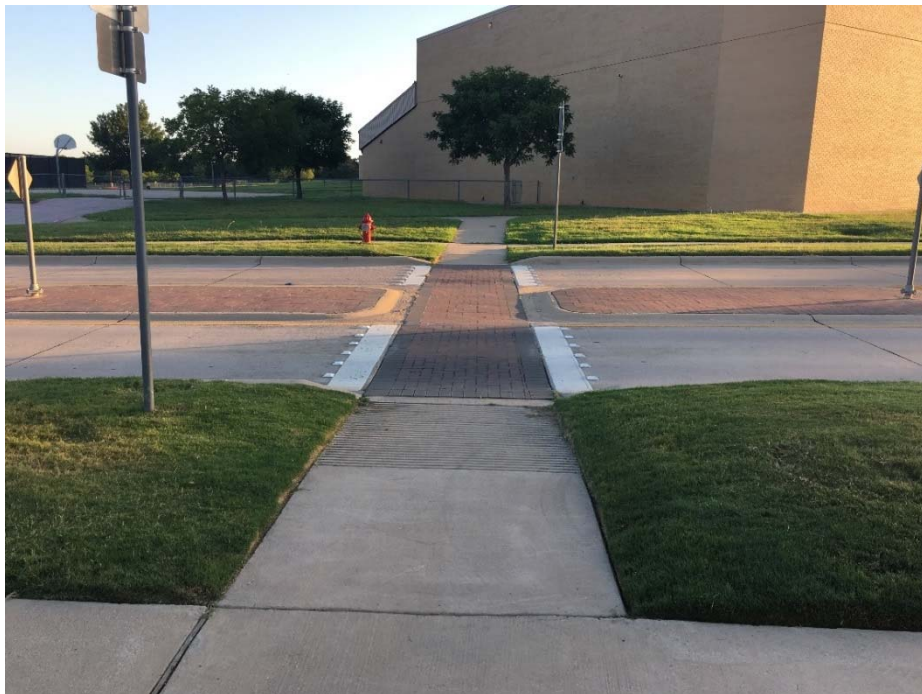
Location 8: Bogart Dr. at west of Hidden Oaks Dr., Looking North
