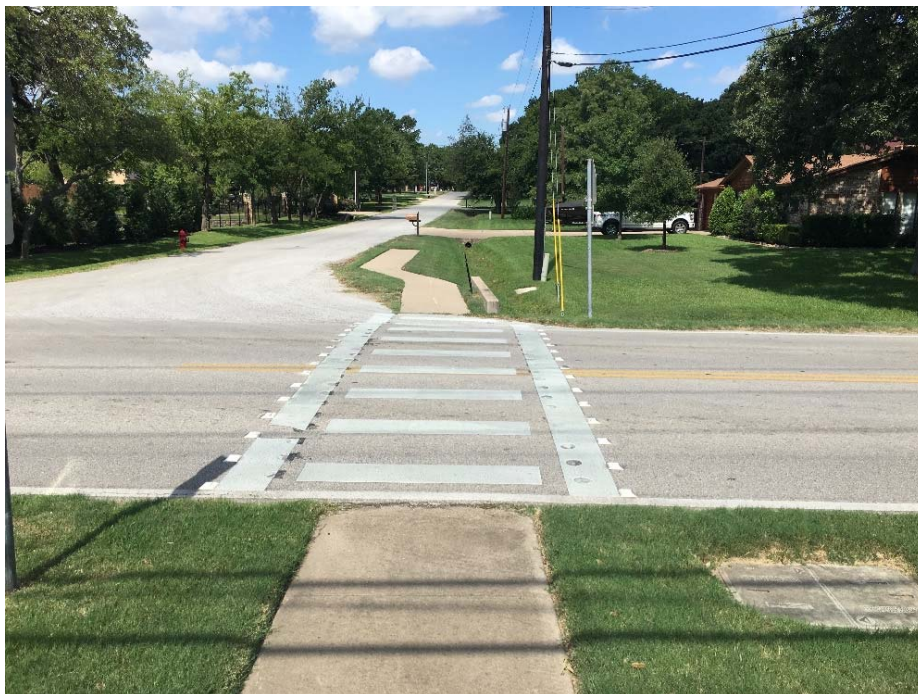
Location 4: Bransford Rd. at Lloyd Cir., Looking West
