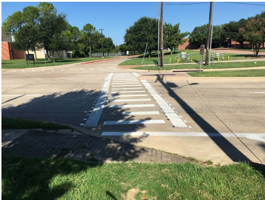
Location 12: Heritage Ave. at Connecting Rd., Looking West
