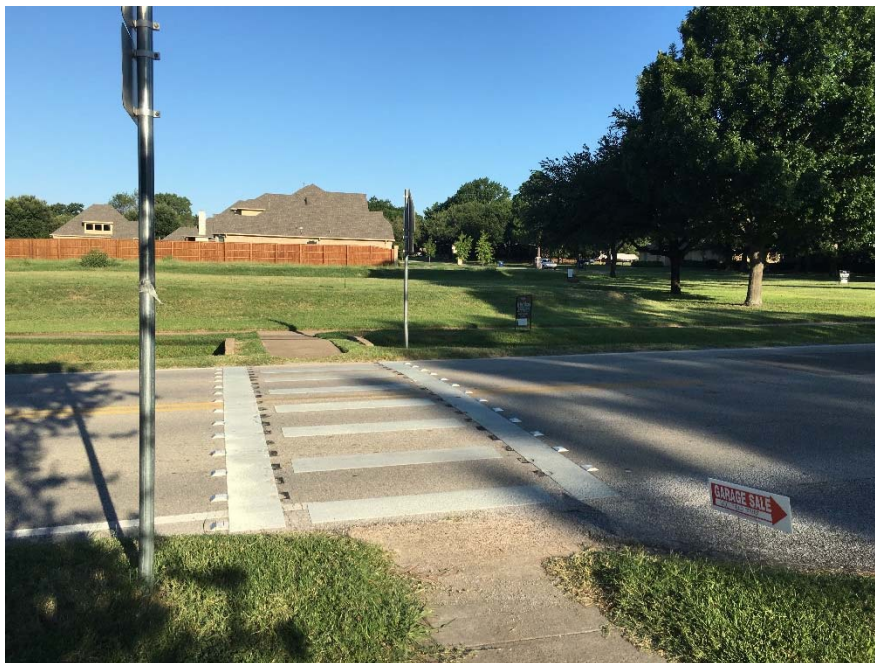
Location 3: Bransford Rd. at Field St., Looking West
