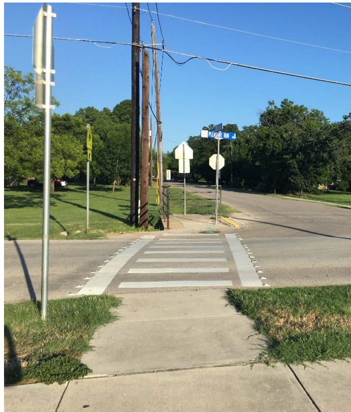
Location 5: Pleasant Run Rd. at Shelton Dr., Looking West
