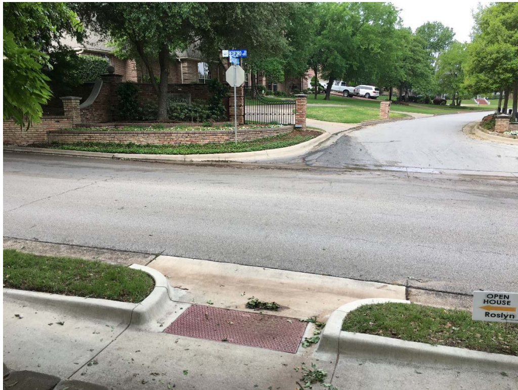
Bedford Rd. at Saddlebrook Dr., looking West
