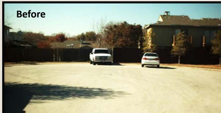
2012 Street Maintenance Project Long Shadow Court – Microseal
