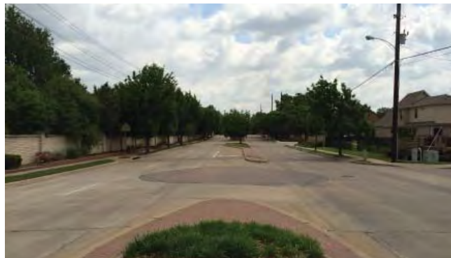
Rebuilt street with additional character elements
