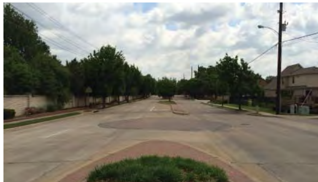
Rebuilt street with additional character elements
