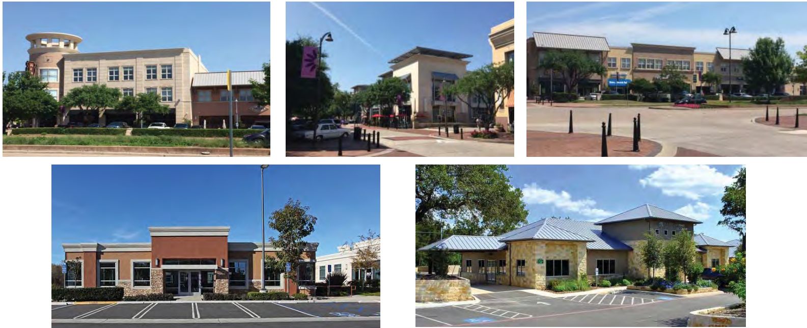
Figure 9.2. Desired Character in the Colleyville Boulevard Corridor
