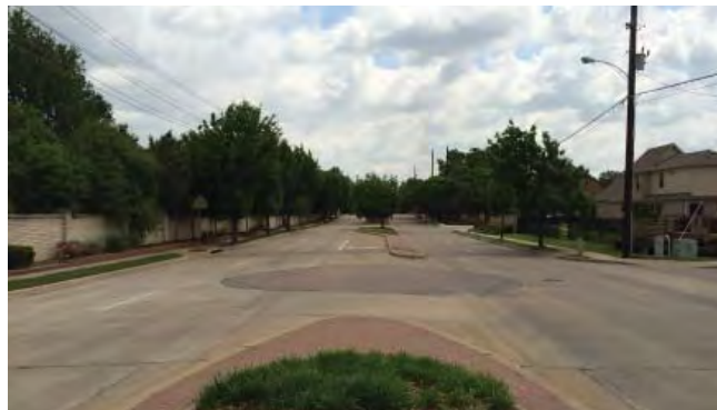
Rebuilt street with additional character elements
