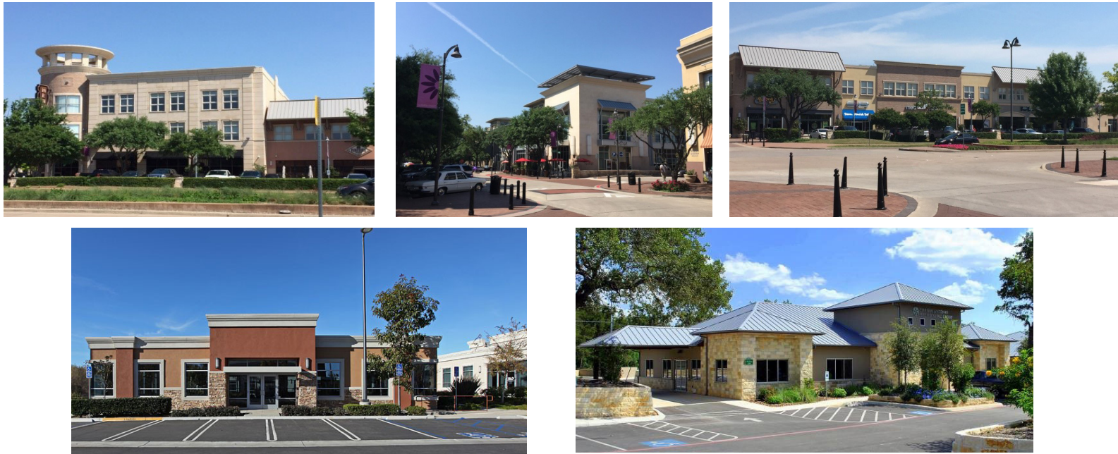
Figure 9.2. Desired Character in the Colleyville Boulevard Corridor
