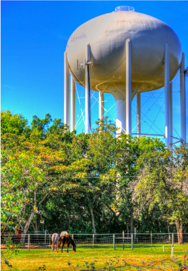
Above is one of three elevated storage tanks located in Colleyville.
