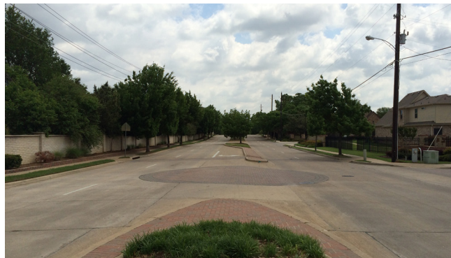
Rebuilt street with additional character elements
