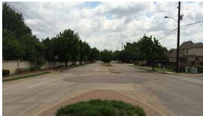
Rebuilt street with additional character elements
