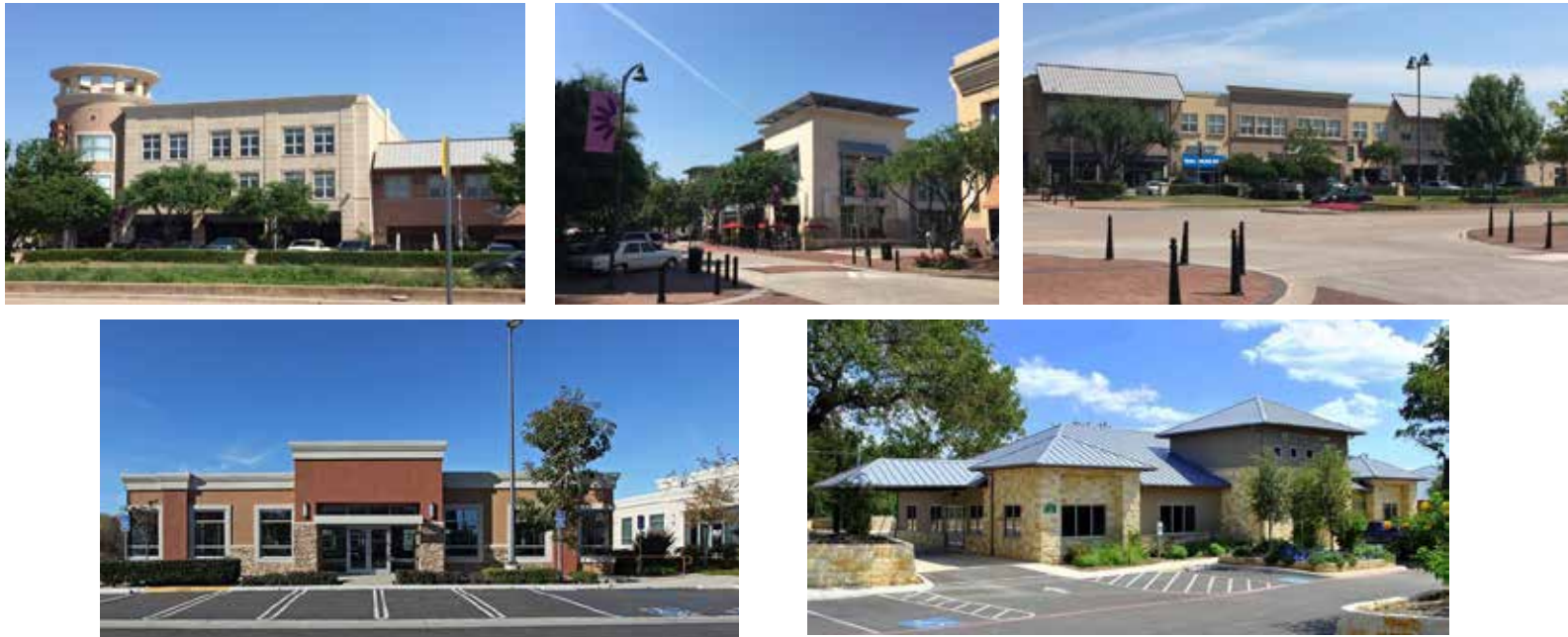
Figure 9.2. Desired Character in the Colleyville Boulevard Corridor
