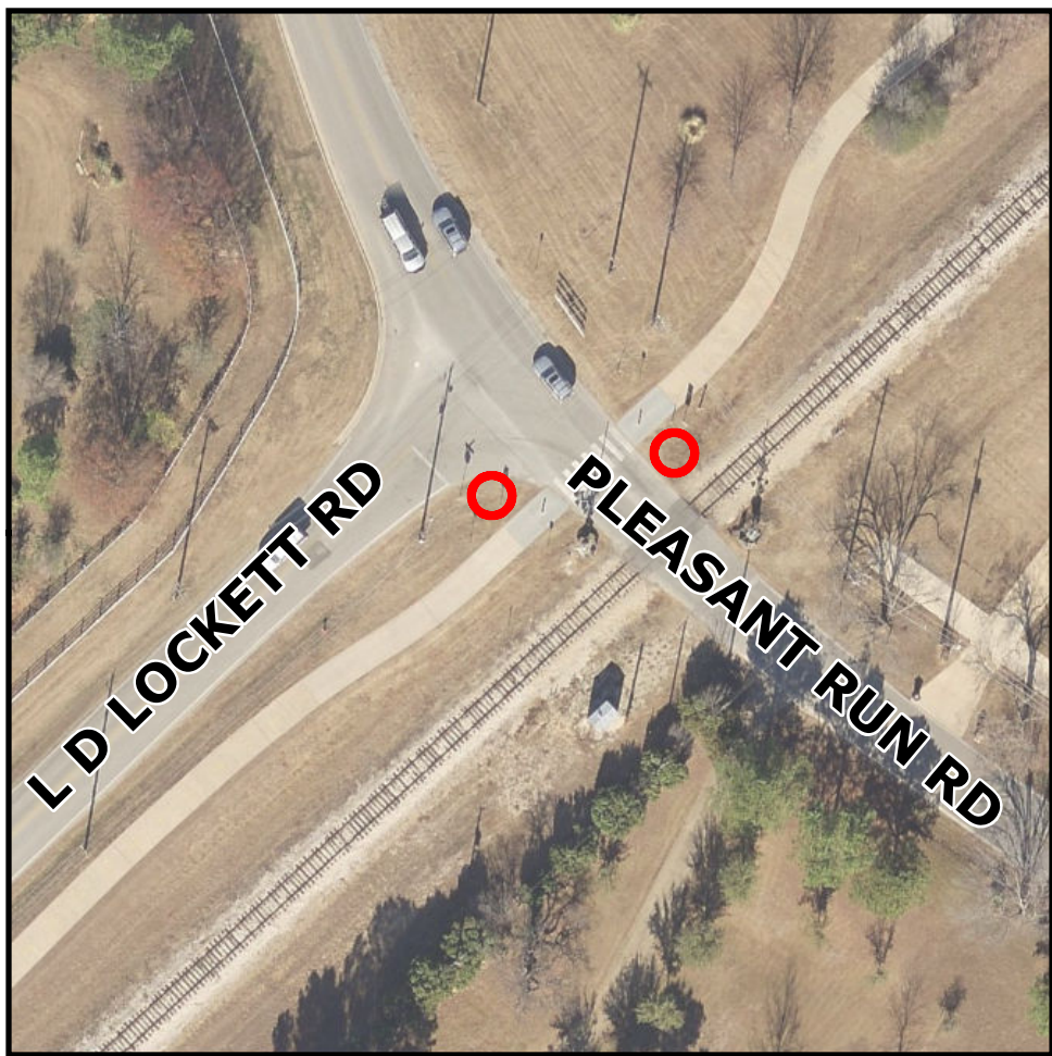
Location 2 Pleasant Run Road at Cotton Belt Trail
