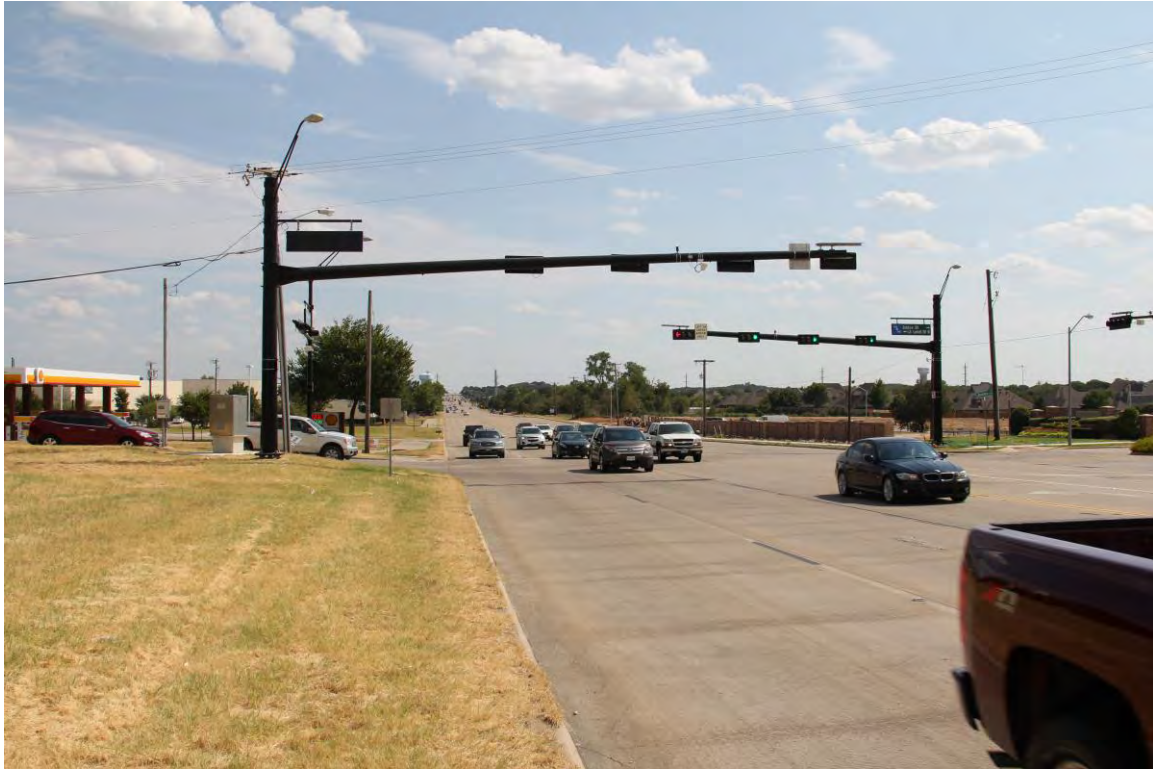
VIEW OF CHELSEA BOULEVARD FACING SOUTH
