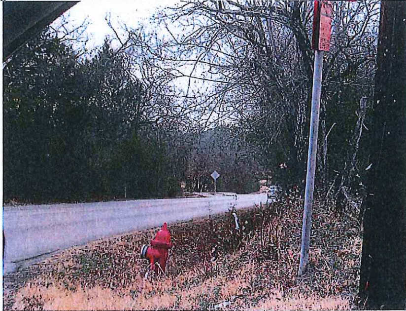
Figure 6: On Bluebonnet Drive Looking West Down Glade Road (SD = 200')
