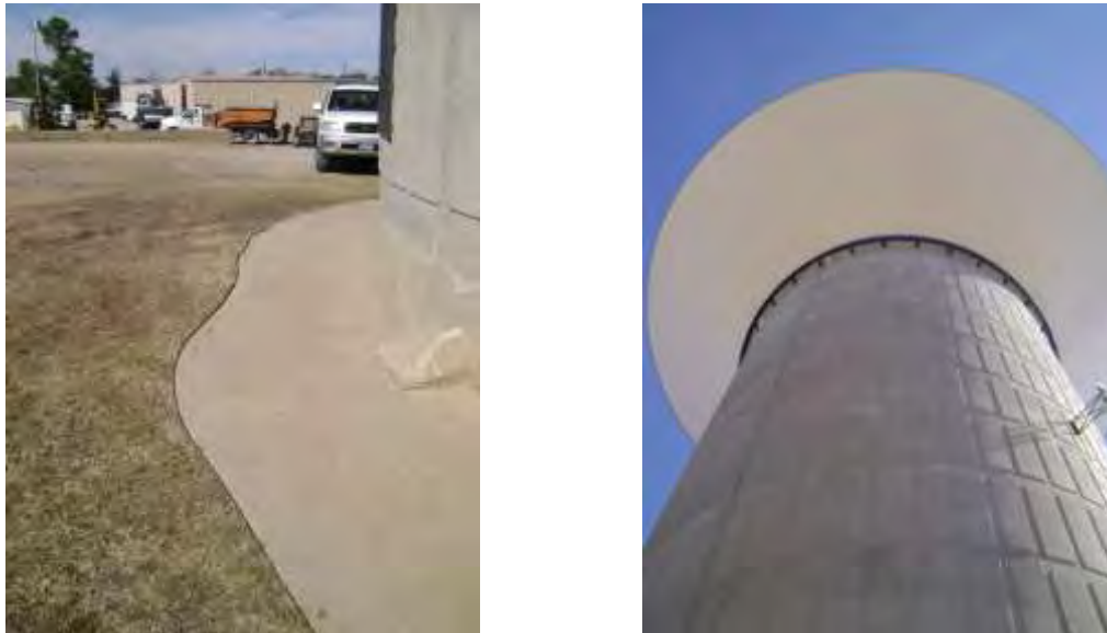
Figure 28: Exterior of Hall Johnson Elevated Storage Tank
