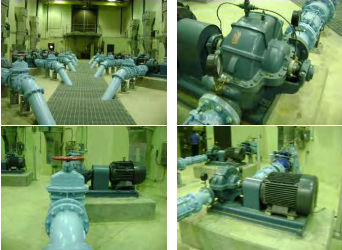
Figure 17: Interior of L.D. Lockett PS Pump Building
