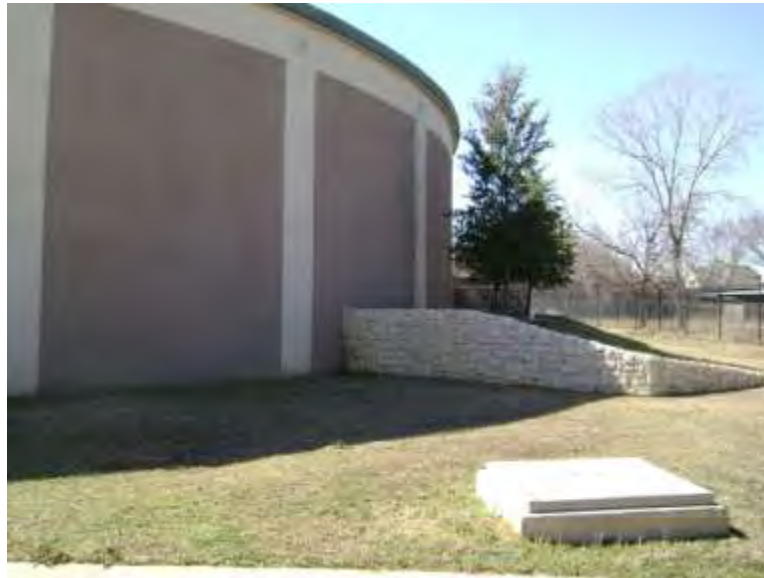
Figure 21: Lockett Ground Storage Tank
