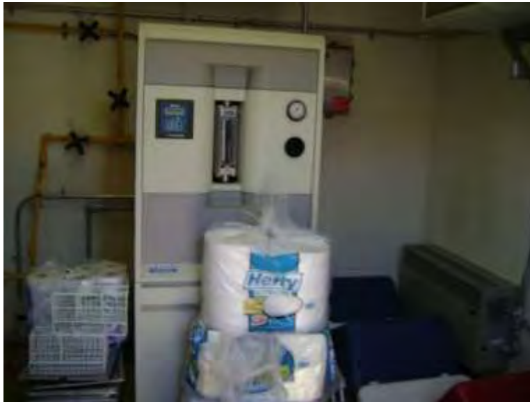
Figure 12: Overland Trail PS Ammonia Building Used for Storage
