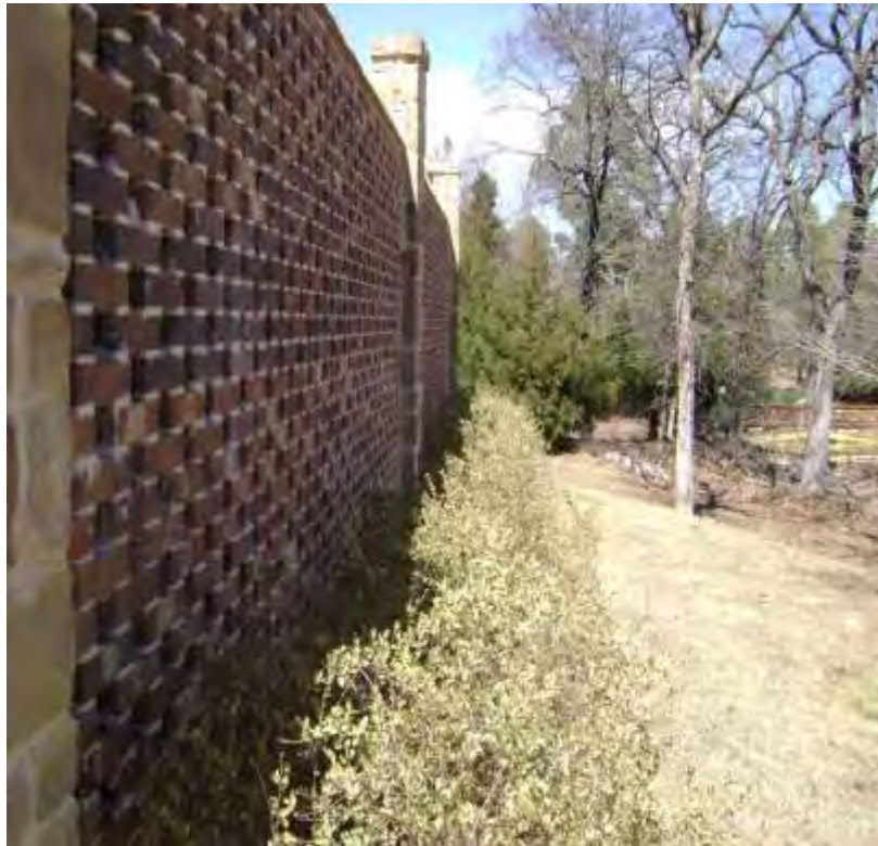
Figure 15: East Fence at Reserve Lift Station
