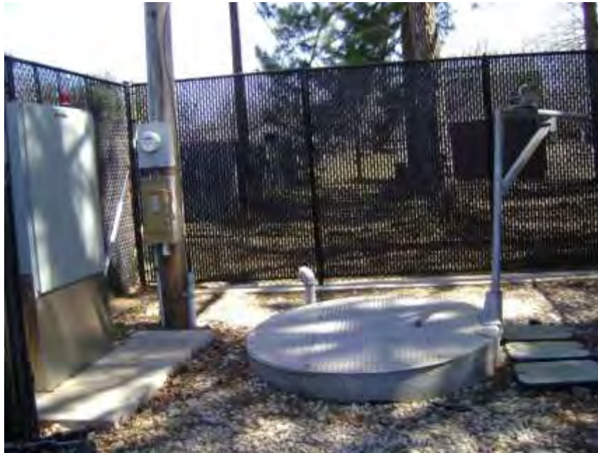
Figure 6: Fencing and Locks at Overland Trail Lift Station
