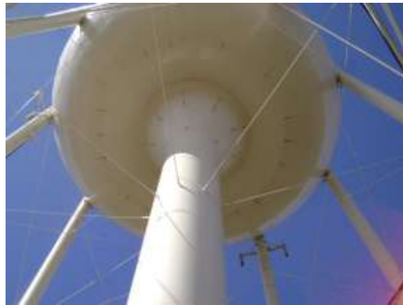
Figure 25: Exterior Coating of Bransford Elevated Storage Tank
