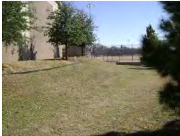
L.D. Lockett Pump Station Site
