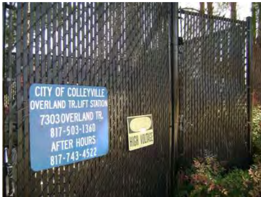
Figure 7: Chain Link Fence at Overland Trail Lift Station
