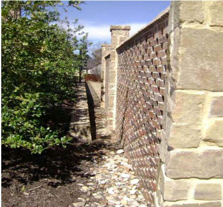
Figure 14: West Fence at Reserve Lift Station
