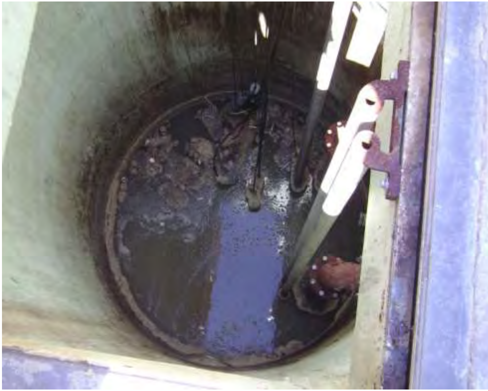
Figure 19: Float and Grease in Wet Well at Reserve Lift Station
