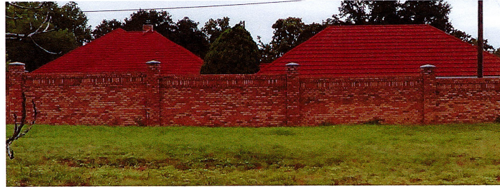
SOUTH PROPERTY ELEVATION TODAY
