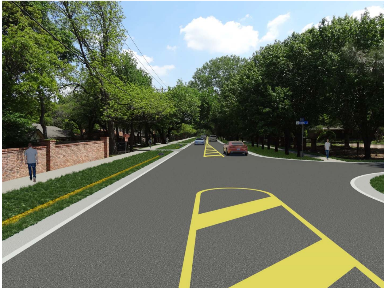
Ribbon Curb with Swale
