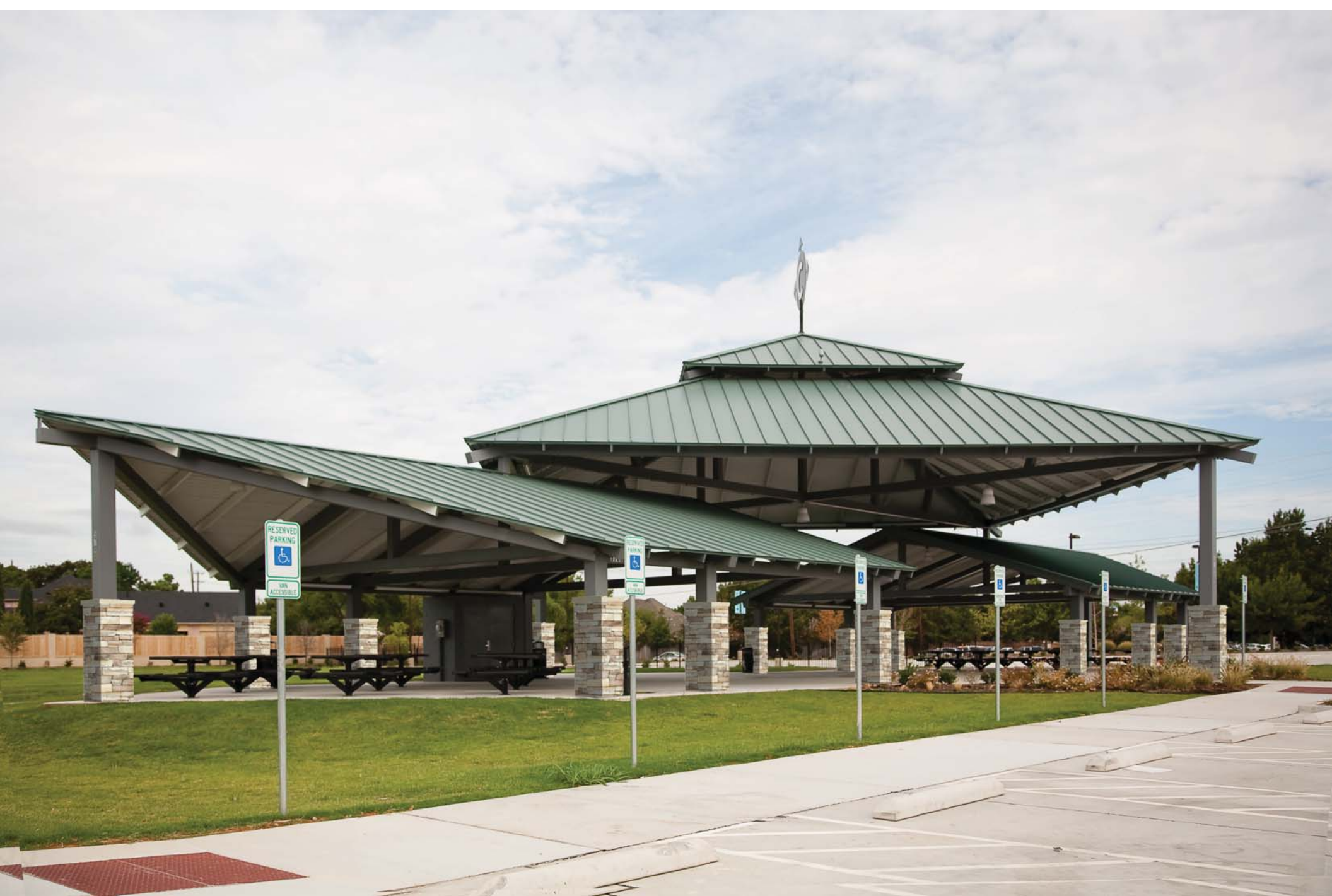
Pavilion Exhibit - Showing Current Columns with Masonry to a Height of Six Feet Only
