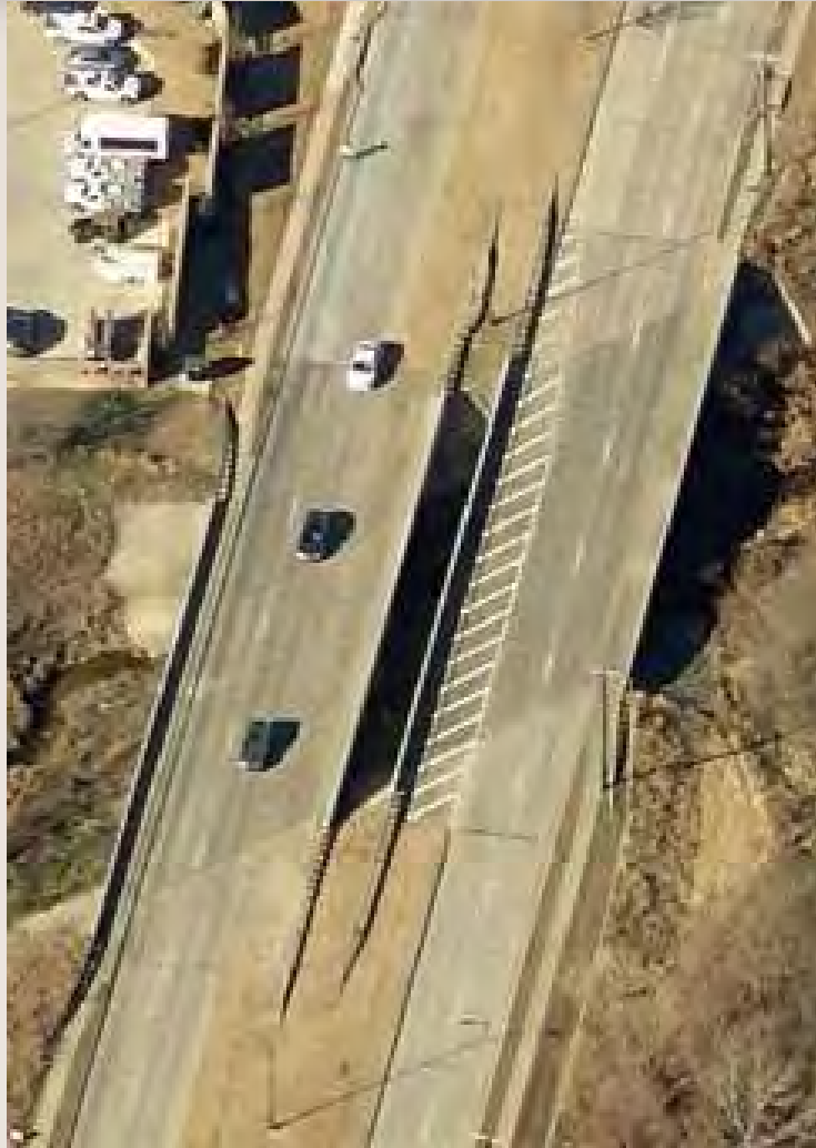
Six Lane Bridge with Four Lanes
