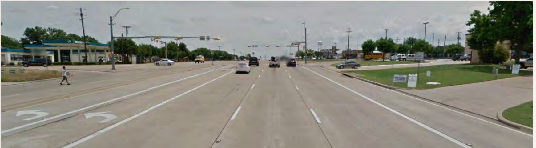
Six Lane Road Heading Toward an Intersection
