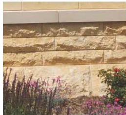
Rough cut lueders limestone w/ cast stone
