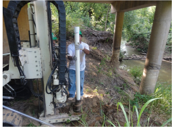
PVC Piping Being Inserted into the First Hole
