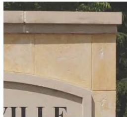
Smooth cut lueders limestone w/ cast stone
