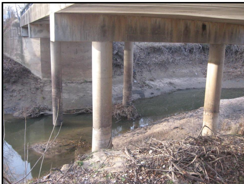
Figure 2 Existing Bridge and Channel (January 2012)
