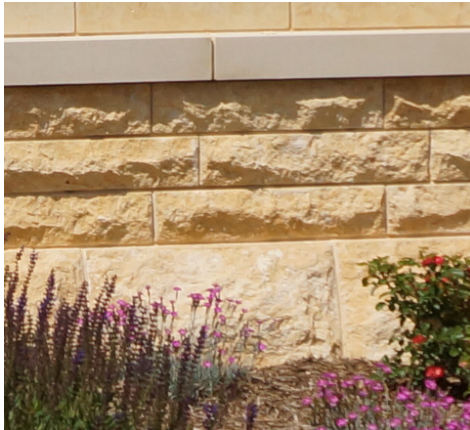
Rough cut lueders limestone w/ cast stone
