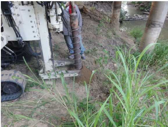
Boring Machine Drilling the First Hole to a Depth 30 feet
