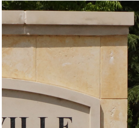
Smooth cut lueders limestone w/ cast stone
