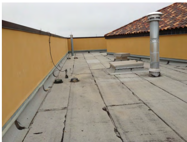
east Roof in good condition needs some maintenance
