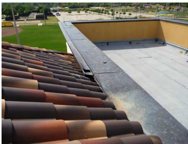
west Roof in good condition needs some maintenance
