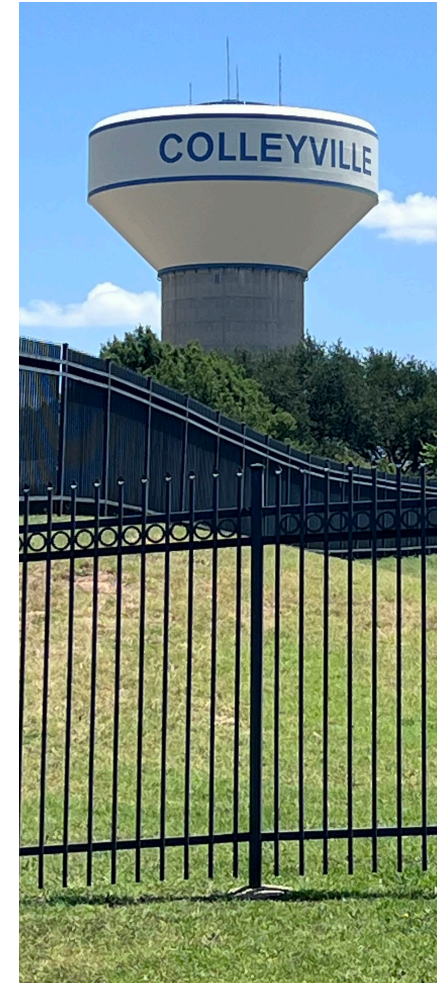
Hall-Johnson Water Tower
