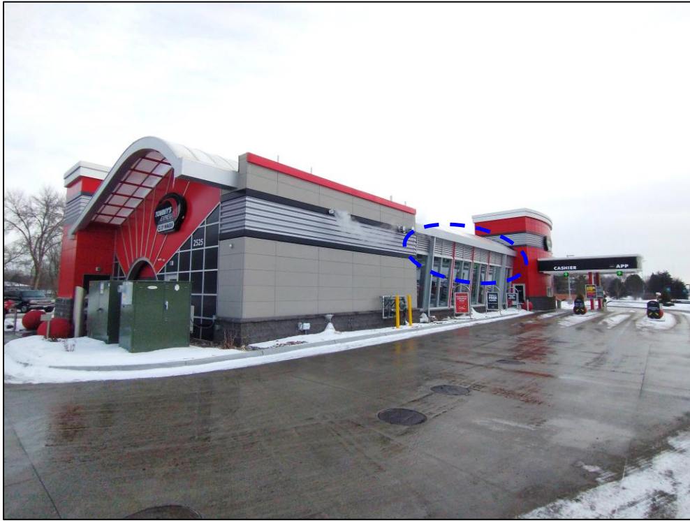
Figure 10 – Photo of the Tommy's Express Car Wash with sidewall louvers circled.
