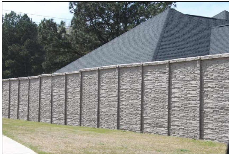
Figure 13 – Hilltop Concrete photo of a concrete fence.
