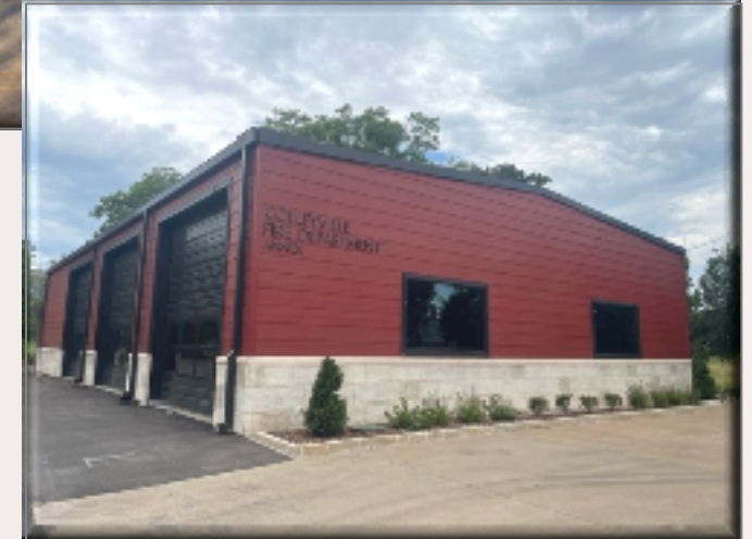
Historic Fire Station Renovation After Costs for Materials and Roofing $176,114
