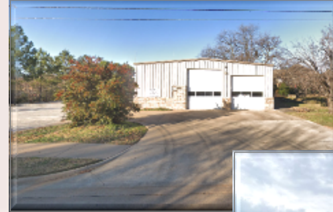
Historic Fire Station Renovation Before
