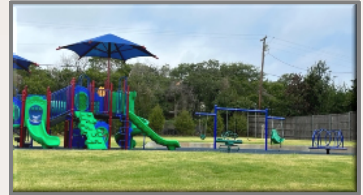
Overland Park Playground with pour-in-place surface, irrigation, grass and trees Contract Amount $208,637
