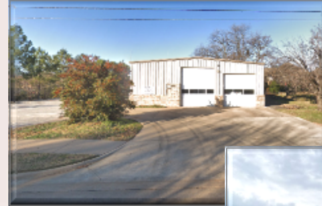
Historic Fire Station Renovation Before
