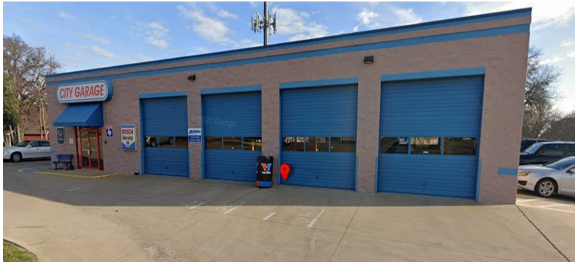
Front of Location
