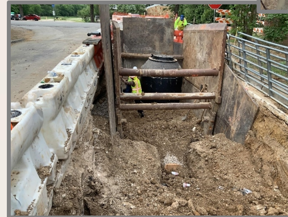
Wastewater Project 5: Quails Path Contract Award $533,111.02
