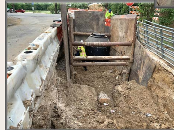
Wastewater Project 5: Quails Path Contract Award $533,111.02
