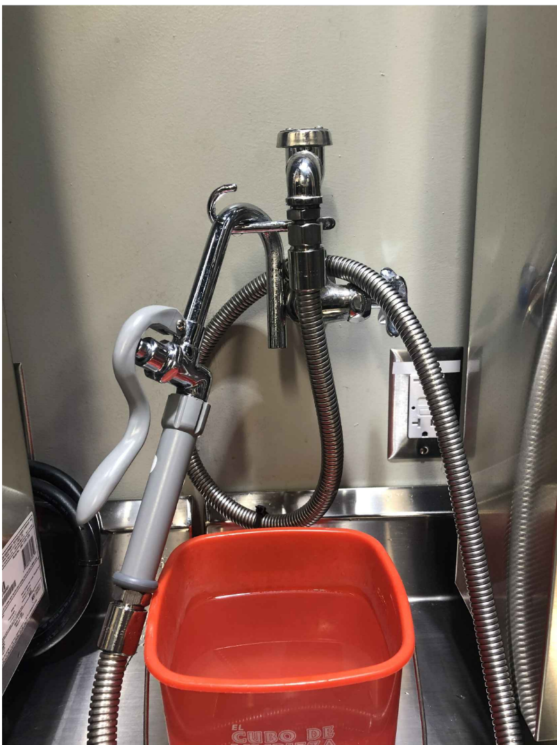
1 JUG FILLER FAUCET COORDINATE WITH PLUMBING DRAWINGS
